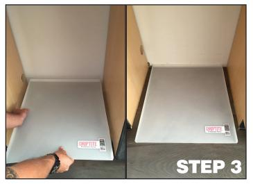
Insert the Dishwasher Pan in the space. Make sure you install the pan approximately 1/2" from the back wall. Use a tape measure to be sure you are centering the pan correctly.
