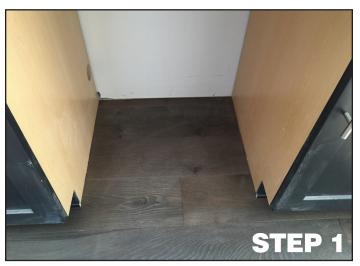
Remove your dishwasher and set it to one side. Make sure to clean up any water or mold from water damage, as well as any debris.
